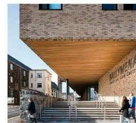
TIMBER SOFFIT TO TERRACES + PODIUM
