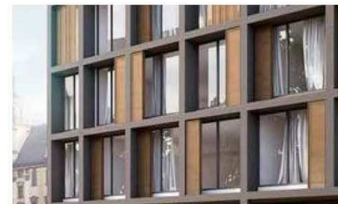
DARK CONCRETE FRAME WITH RECESSED GLAZING + SCREEN
